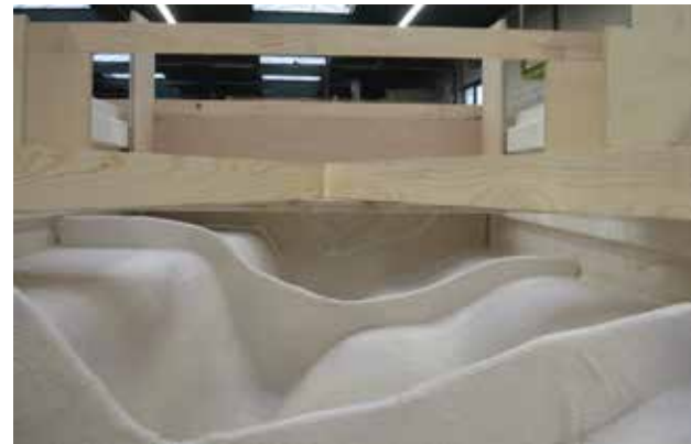
Further interior stiffening of laminate and 18 mm plywood strips connected
