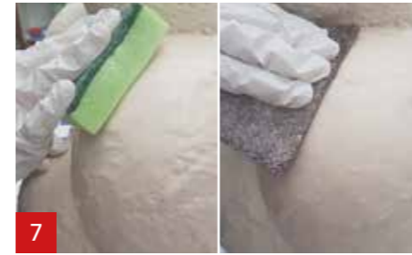
7 Or use (after ±20 minutes) a damp sponge or a waterproof sanding pad.
