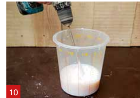
10 Put the mixer (skew) in the A1 Liquid cup and create a swirl.
