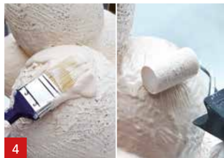
4 The A1 can be applied with a: brush, roller, spatula or squeegee.
