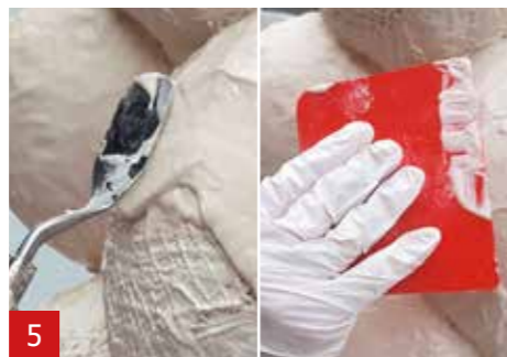
4 The A1 can be applied with a: brush, roller, spatula or squeegee.
